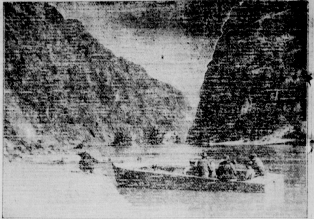
Party of Government engineers inspecting Boulder Canyon dam site on the Colorado River where it is proposed to erect the world's largest flood control dam. The project is unique in that it is to be financed entirely from the water and hydro-electric power it will make available.
