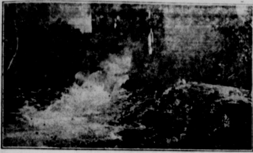
2,000 gallons per minute irrigation well near Lockney
