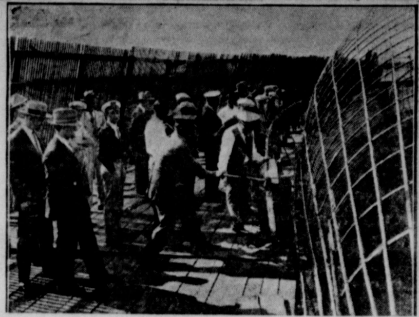
NEW ALL METAL DERIGIBLE UNDER CONSTRUCTION AT GLENDALE, CALIF.
