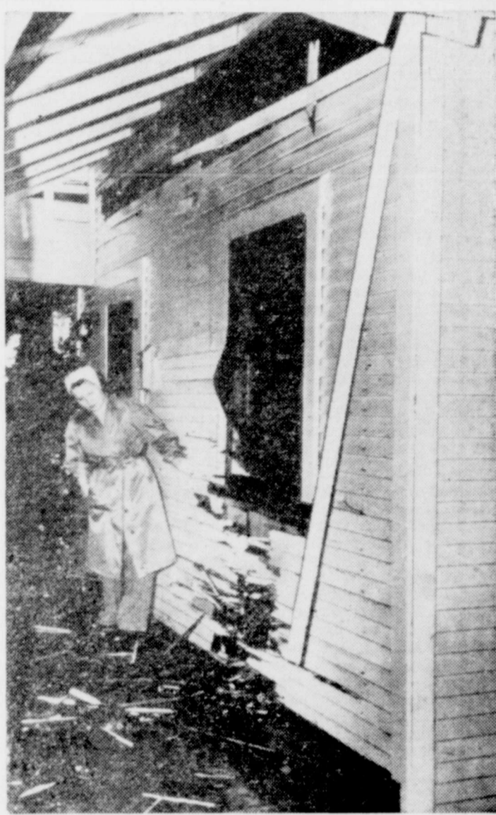
NON-STRIKER'S HOME BOMBED —Mrs. William J. Saltis, wife of a non-striking motion picture studio machine shop foreman, inspects damage done to their home when a crude bomb exploded under bedroom window. This and another similar bombing in Los Angeles were ascribed by police to zoon squads.
