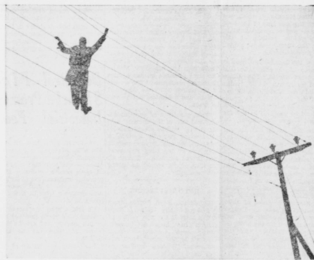
THE HARD WAY —This British Post Office linesman does a bit of wire-walking near London as he repairs telegraph wires damaged by a storm along the road between Bude, North Cornwall, and Holsworthy, Devon, England. Many an ex-GI traversed this road during his stay in England.
