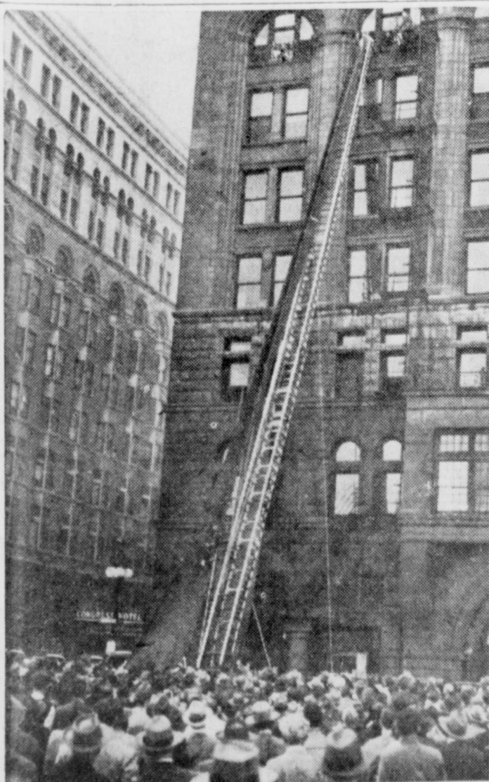
SAFETY CHUTE —Chicago firemen demonstrate the new safety chute. Made of canvas, the long slide is used to quickly remove persons from burning buildings to safety. Here a fireman is catapulted from the seventh floor.
