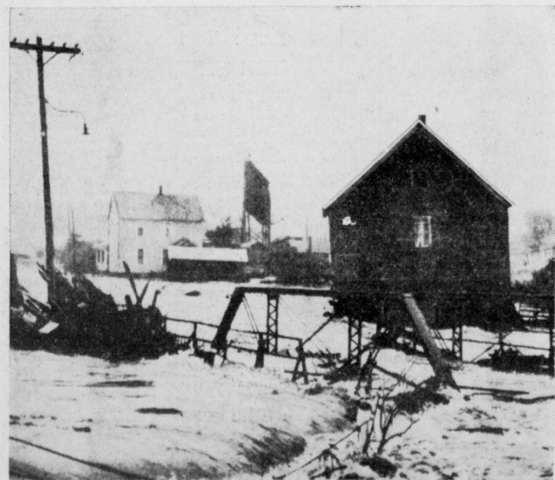
HISTORY MAKING FLOOD —One-seventh of the people in Mellem, Wis., were left homeless as the Bad River sweeps on, destroying town after town in upper Wisconsin. Here the raging waters submerge a bridge at Mellem.
