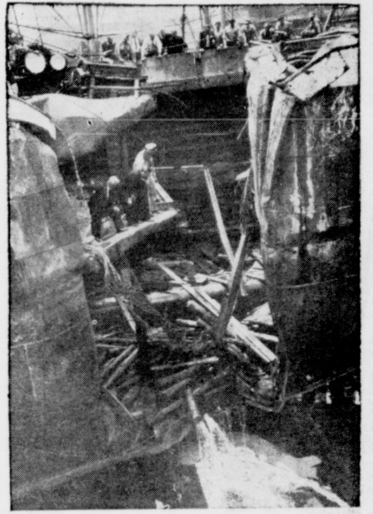
MADE IT—After having a giant hole ripped in its side by the tanker Amiens, off Barnegat Light, the Royal Netherlands cargo ship Tiberius was brought into Brooklyn shipyard. Here, dock workers examine the badly damaged Tiberius.
