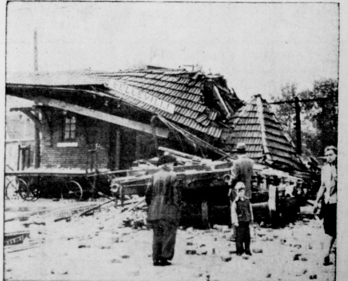
NO ONE WAS HURT in this unusual railroad accident at Belleville, Ill., that miraculously caused only property damage. Wreck occurred when three flatcars were derailed from a passing freight train due to a faulty wheel flange.
