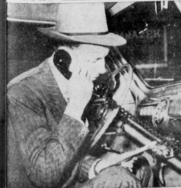
HELLO, CITY DESK—In first public use of automobile telephones, Richard Everett of the St. Louis Star-Times calls in his story from his car on outskirts of city. Telephones is plugged into auto radio which broadcasts to telephone company system, which, in turn, dials number requested.
