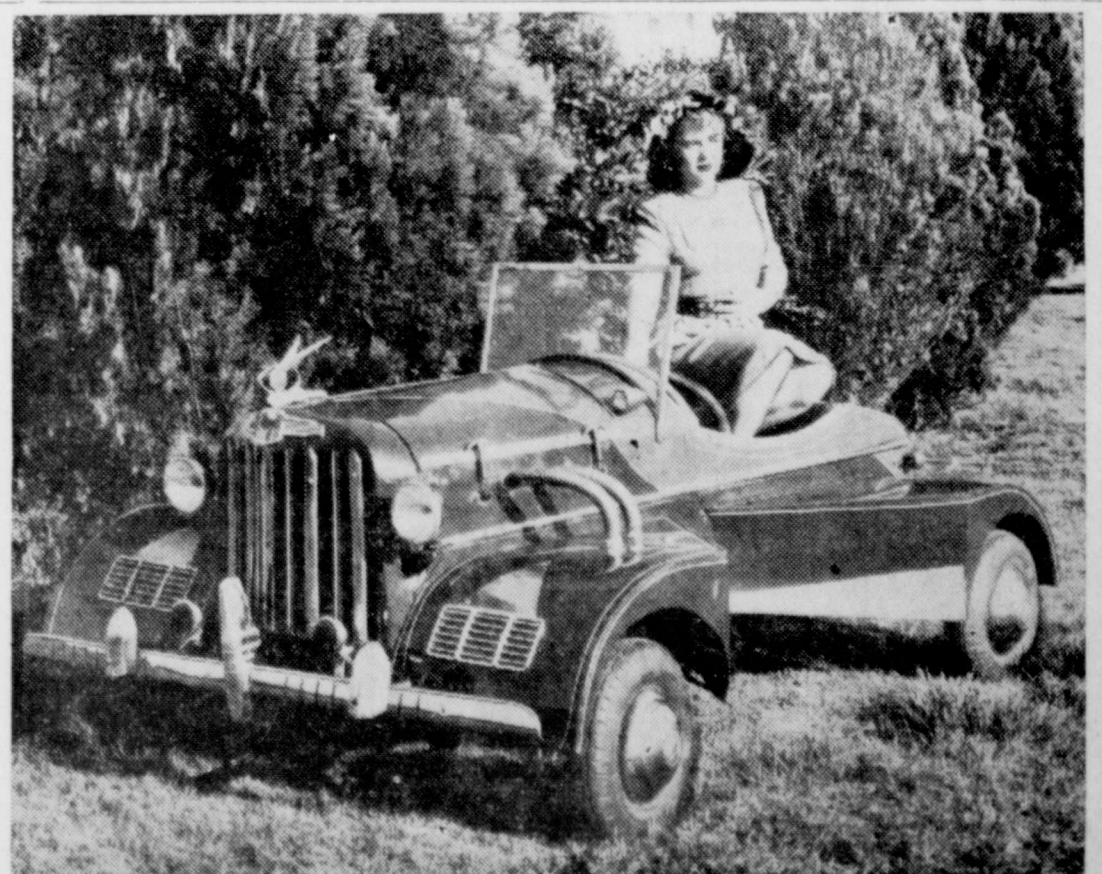
WANT A CAR? MAKE IT YOURSELF —Emory Kent, Wichita Falls, Tex., mechanic, made this automobile for his daughter, Helen, 14, out of discarded parts. It goes 50 mph, gets 55 miles per gallon of gasoline.
