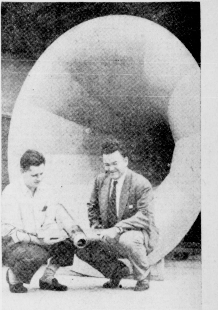
AND STILL MORE SPEED —University of Southern California engineers, Robert T. DeVault, left, and R. E. Marquardt, examine model of jet motor which they hope will develop 1,000 to 2,000 mph speeds. In background is wind tunnel used for testing.
