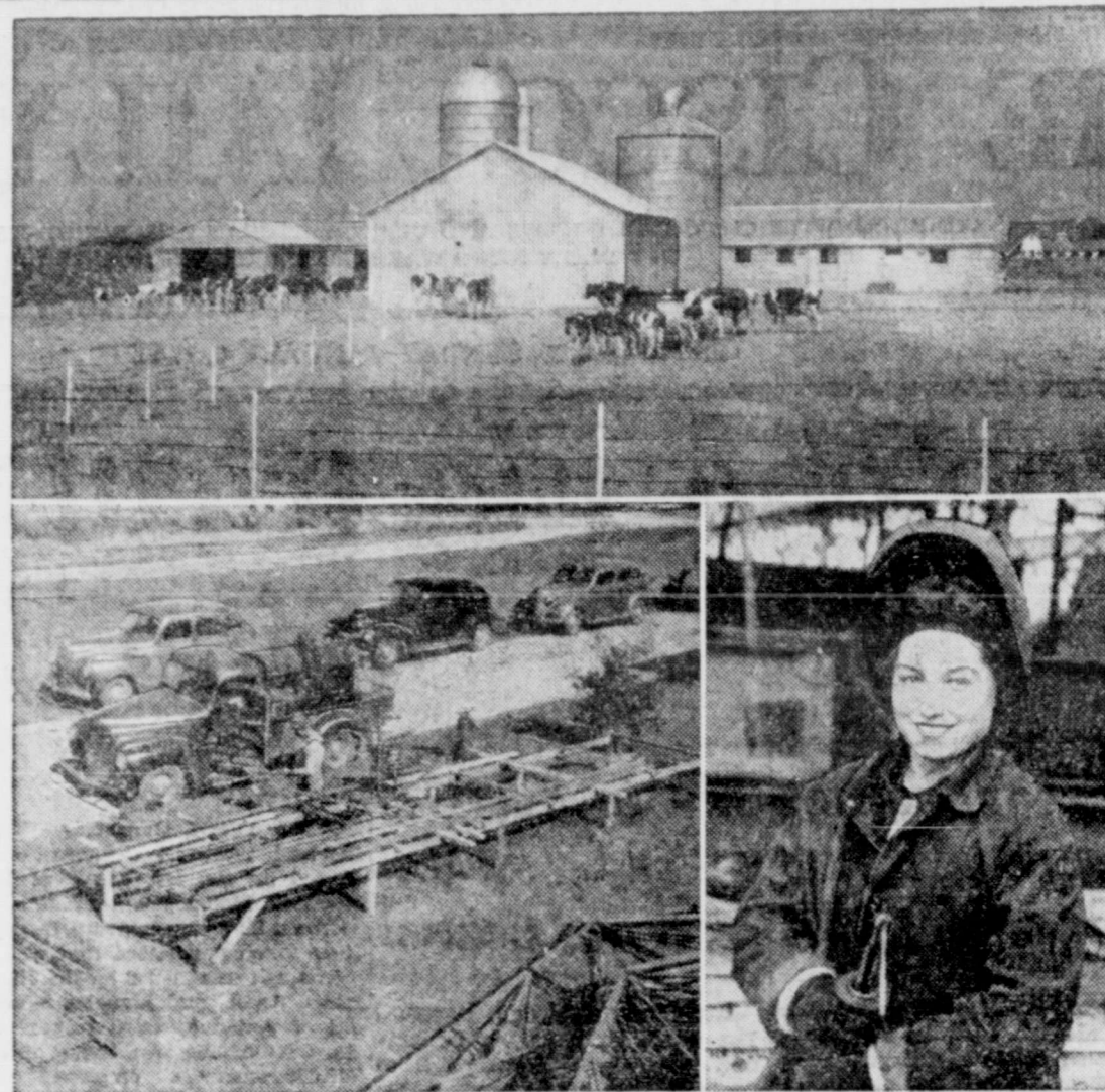
THIS GIRL WELDER was pleased as punch when she learned her job to help win a war. She may smile again at the opportunity to apply her skill in welding structural members for farm buildings on the site, a new and lighter job created by a new system of construction developed by research engineers of Carnegie-Illinois Steel Corporation, U. S. Steel subsidiary, and University of Wisconsin. This steel development also promises work for the HANDY MAN AND HIS TRUCK, be he honorably discharged soldier or a temporarily displaced war worker. The SITE-WELDED FARM BUILDINGS (above), with their shining steel sheathing, promise low-cost help toward the solution of two vexing postwar problems—shortage of building labor and of traditional structural materials.
