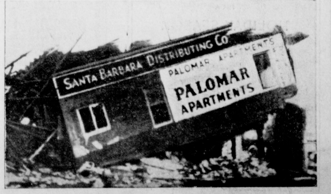
APARTMENTS WRECKED BY BLAST —When a truck carrying butane gas for a bottling plant blew up, it left this wreckage of a 20-apartment building at Santa Barbara, Calif. Five persons were killed in the blast, which also destroyed the bottling plant. Building was completely ruined.
