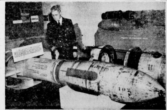
MEET "THE FRITZ"-Secret German FX 1400, a remote control, free-falling bomb is examined by Commo. H. A. Schade, Director of Naval Research Laboratory. Bomb, known as "The Fritz". weighs 3000 pounds, is armor-piercing and has no propulsion unit. It can be guided by radio.
