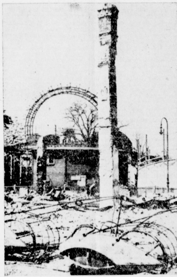
AMUSEMENT PARK —This one, wobbly chimney and the twisted remains of a ferris wheel and high-swing ride are all that remain of this Viennese amusement park. Park was hit by American, Russian and German shells and bombs.
