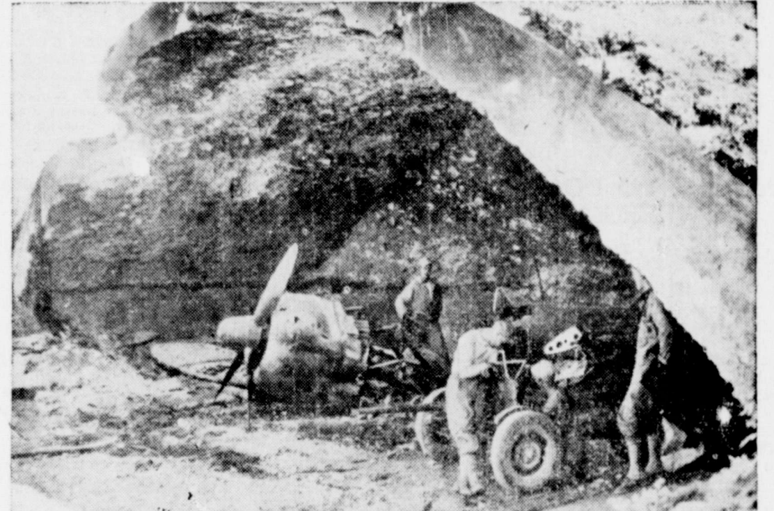
BANKING THEIR SHOTS —Heavy concrete revetment on Jap airfield on Okinawa failed to protect enemy plane cached there. American gunners banked one of their shots and scored direct hit. Here Marines examine demolished plane. They are using shelter as anti-tank gun position.
