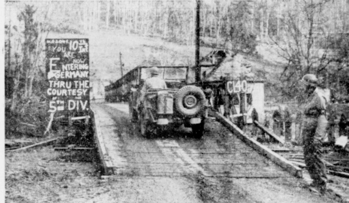
OVER-THE-LINE in Germany is marked by sign informing all who cross that they do so by courtesy of the 5th Division. Here jeep crosses bridge spanning Sure River in wake of 5th Div. advance into Naziland. Military policeman stands at one side. (Acme Photo by Charles Haacker for WPP.)
