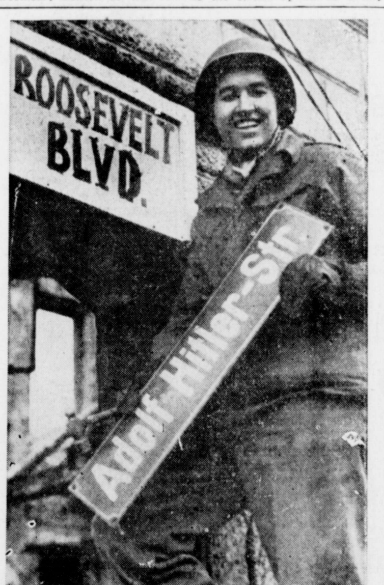
NEW ORDER—S/Sgt. George A. Kaufman of Fort Smith, Ark., removes outdated Adolf Hitler Strasse sign for more appropriate Roosevelt Boulevard designation. Smiling Yank in Kreifeld is with Signal Company of 9th Army unit that captured Nazi town.
