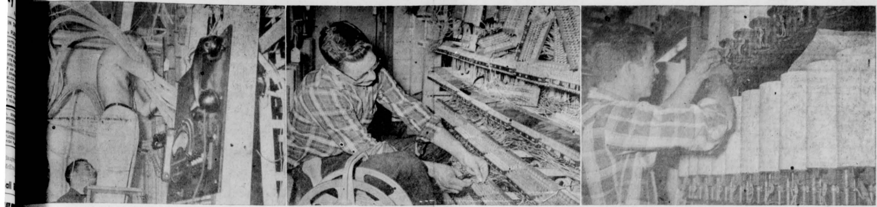
A technician helping to install West Texas Telephone Company's dial system is not carrying that mass of wire anywhere—he's just holding onto it works on some of the dialing equipment. Joe Thornberg of Indianapolis, is watching Horn, who is from California.
