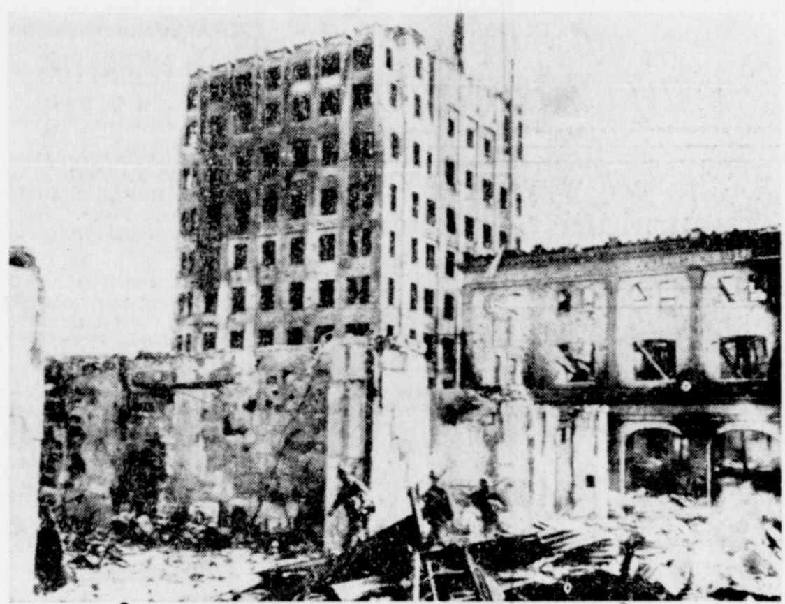
TYPICAL MANILA SCENE—Portraying Jap ruthlessness, this building in the heart of Manila's business section is unrepairable after retreating enemy set it ablaze. Japs are pillaging, destroying and burning everything in sight as Americans push them south. Here Yanks go through ruins.
