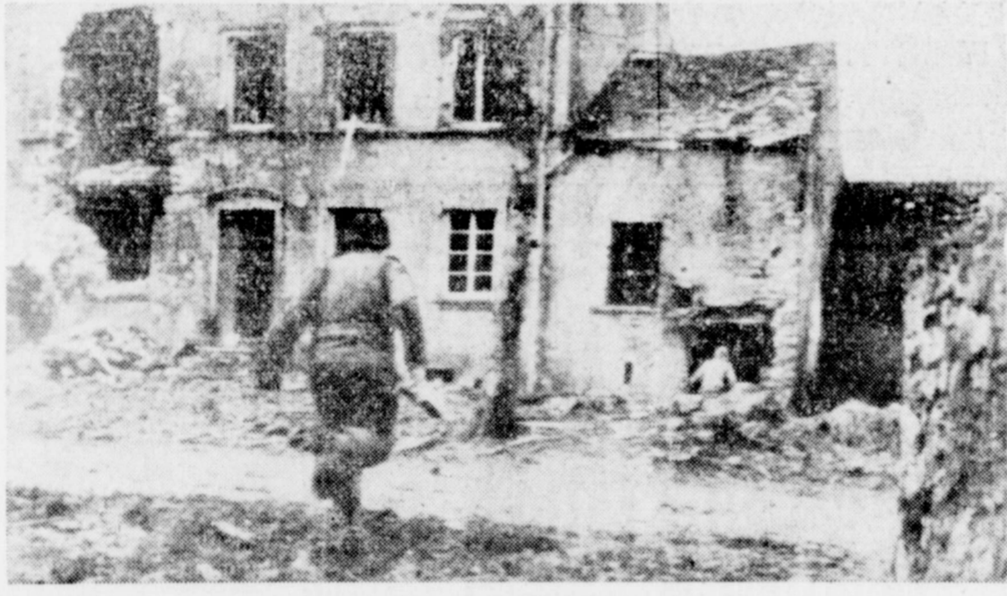
DASHING FOR COVER—Combat infantryman of the Third Army runs for shelter in wrecked building. His companion is already entering bomb crevice during height of enemy fire in battle for Sinz, Germanv. Strewen debris shows fury of combat. (U. S. Signal Corps Photo.)
