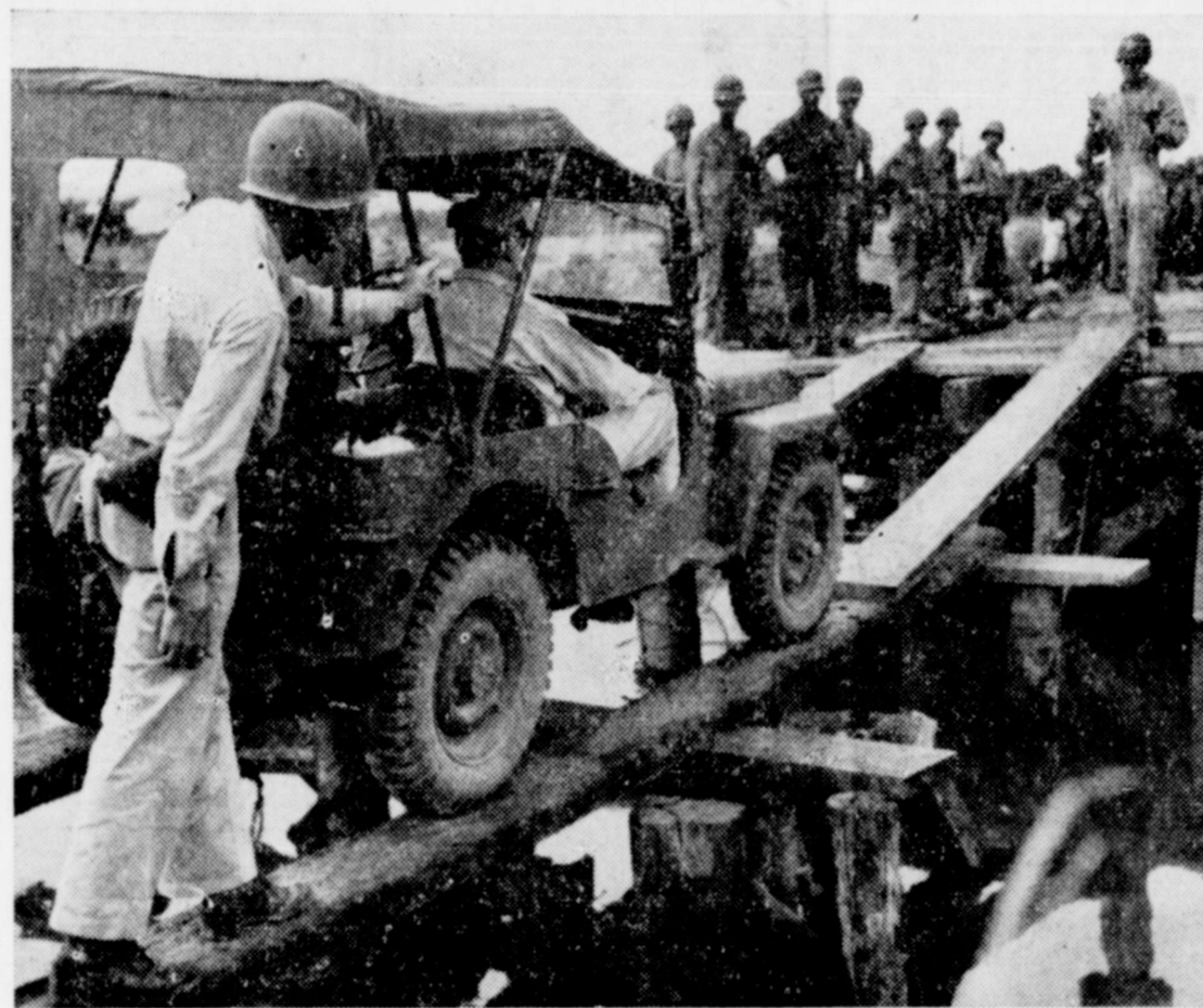
CAREFUL NOW —Gen. Douglas MacArthur sits coolly in seat as jeep starts on precarious crossing over rickety bridge at Camiling on Luzon. Yank in foreground guides vehicle with firm hand while soldier in background gives "come-on" signal. Planks were hastily stretched across bombed-out bridge to permit general's crossing.
