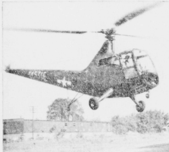
SOMETHING NEW —With straight up take-off, first helicopter built by a Detroit manufacturer makes initial test flight from plant's airport. This marks successful application of automotive assembly line technique to mass production of new-type aircraft.
