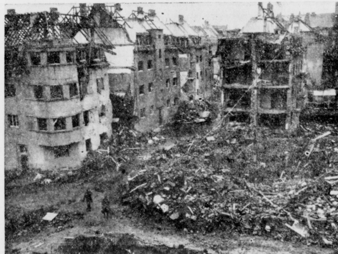
ACHING AACHEN—Guttered houses, broken masonry and concrete litter streets of Aachen-Fort, about 150 yards from Nazi stronghold of Aachen. Surbur already in American hands and GI's are continuing battle for the city proper with fierce assaults. Already they hold half of it.
