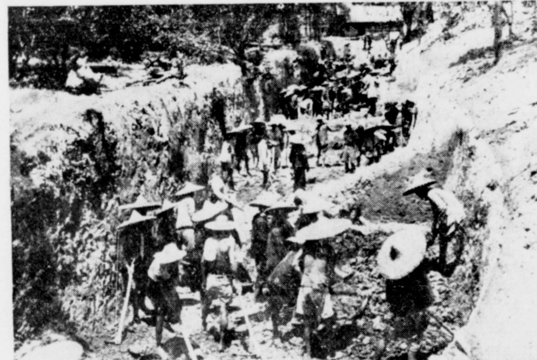
DIGGING IN—Coolie laborers work earnestly in preparation for defense of Kweilin, Jap objective in Southern China. Here they dig deep trench to help stop enemy, reported to be within 80 miles of city.
