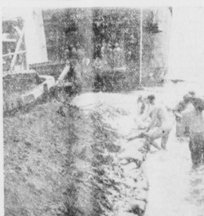
ENGINEERS AT WORK—Preparing ramp to enable landing craft to unload supplies on beach at Sarmi, Dutch New Guinea, is unit of Army Amphibious Engineers. Nude and near nude they work in hot sun. Fighting men know that without support from these men invasion landing operations would be almost impossible to fulfill.
