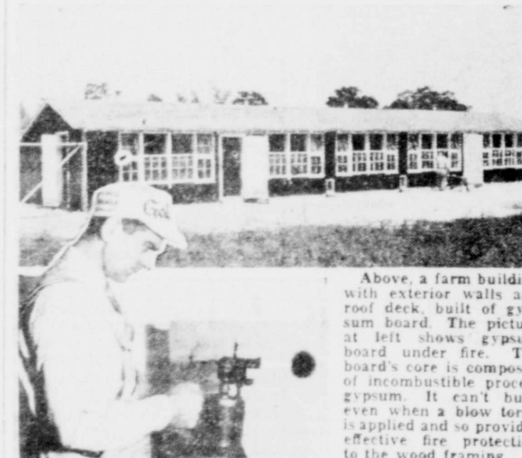
Above, a farm building with exterior walls and roof deck, built of gypsum board under fire. The picture at left shows gypsum board under fire. The board's core is composed of incombustible process gypsum. It can't burn even when a blow torch is applied and so provides effective fire protection to the wood framing.
