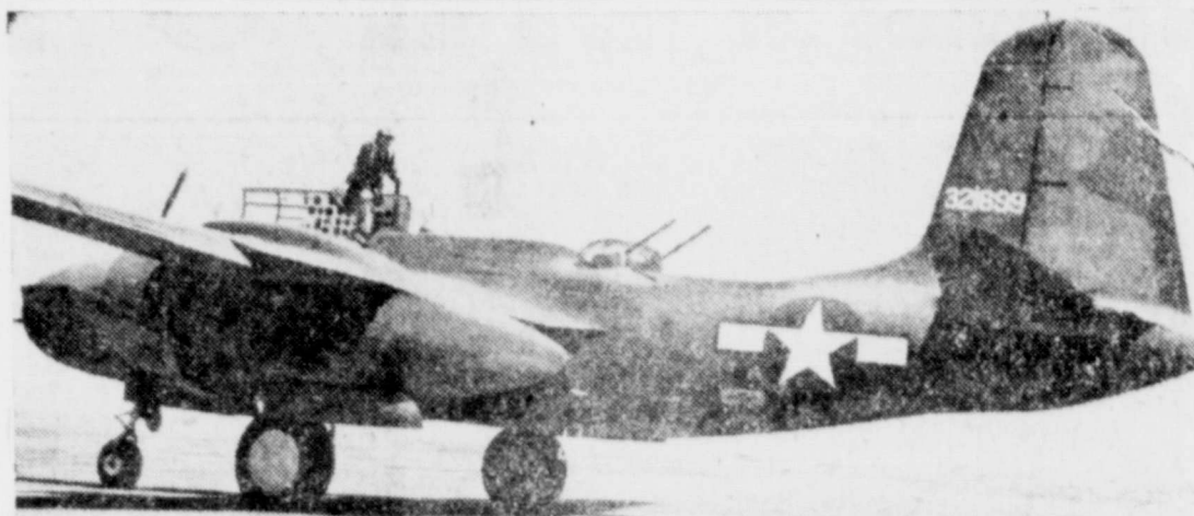
NEW ADDITION—Two more 50 caliber machine guns in a power turret are latest addition to Douglas A-20 Havoc, just off assembly line at Santa Monica, Cal. Army reveals that bomber now carries nine heavy machine guns for pulverizing the enemy.
