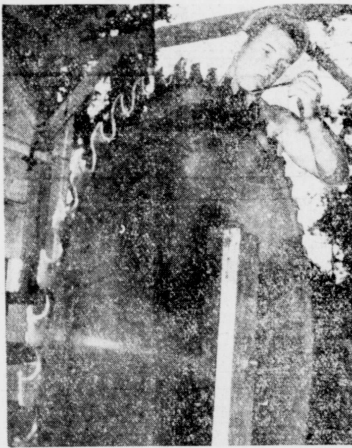
BOUGAINVILLE BUZZ SAW—Army engineers on Bougainville have set up a lumber mill to supply wood for buildings, bridges and any installations required. Here, Cpl. Frank Daly of N. Y. sharpens up the teeth of a four-foot circular saw.
