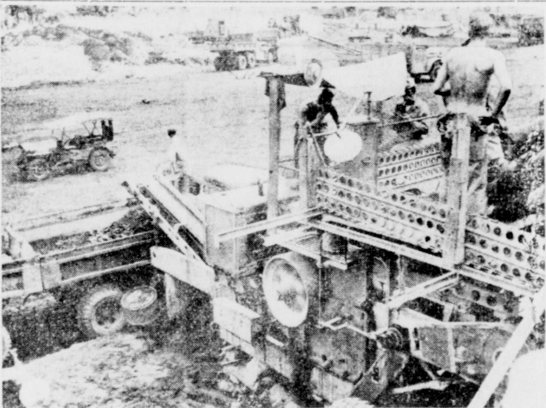
ROCK CRUSHER—Army engineers set up rock-crushing equipment on Cape Gloucester airport, "oon after Marine invaders wrested strategic New Britain field from Japs. Rock crushers provide enough solid surface for reconditioning airfield. (U. S. Marine Corps Photo.)
