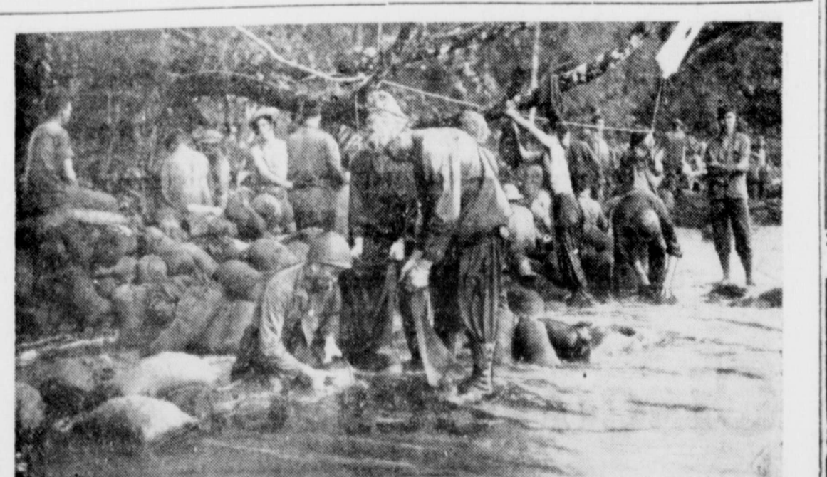
OUNCE OF PREVENTION—Battle-wise Marines know from experience that wet sand is good protection against enemy bullets. Photo shows Leathernecks just after landing on New Britain, near Cape Gloucester, scooping up sand to fill bags for barricades.
