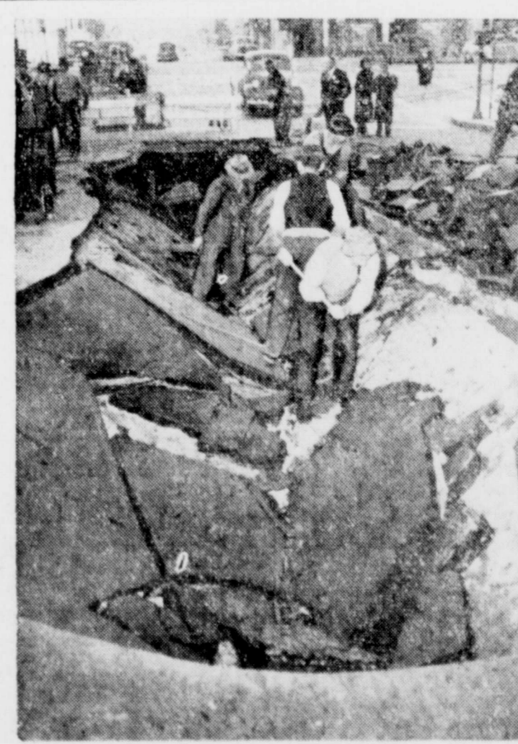
STREET SCENE—Now you see it, now you don't. San Franciscans were surprised when what appeared to be perfectly good sidewalk disappeared from view with a roar. Cave in occurred when broken water main washed away soil under pavement.
