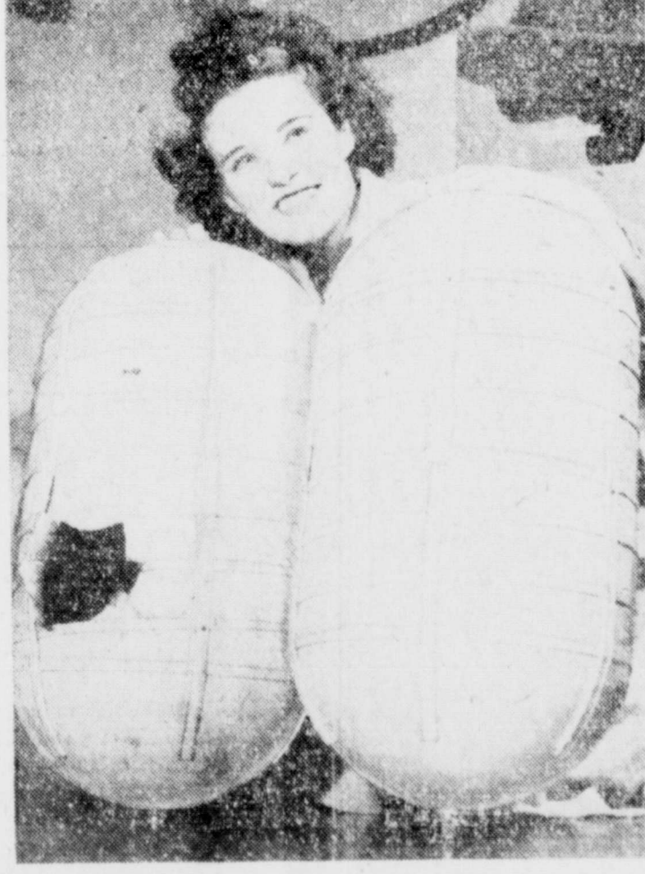
SHATTERPROOF—Cylinders carrying compressed oxygen no longer explode when struck by machine gun bullets. Mrs. Glory Wuchter of Chicago shows cylinder at left, which tears instead, owing to second weld at seams of tanks. Harper's to crew is broken.
