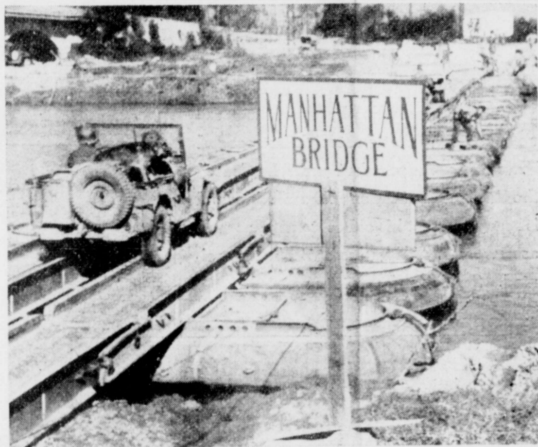
JUST LIKE HOME—Any similarity to New York's Manhattan bridge is purely coincidental, but Yanks in Italy couldn't resist the gag. Trucks and jeep speed across Voltorno on ponton bridge and resume road on other side.
