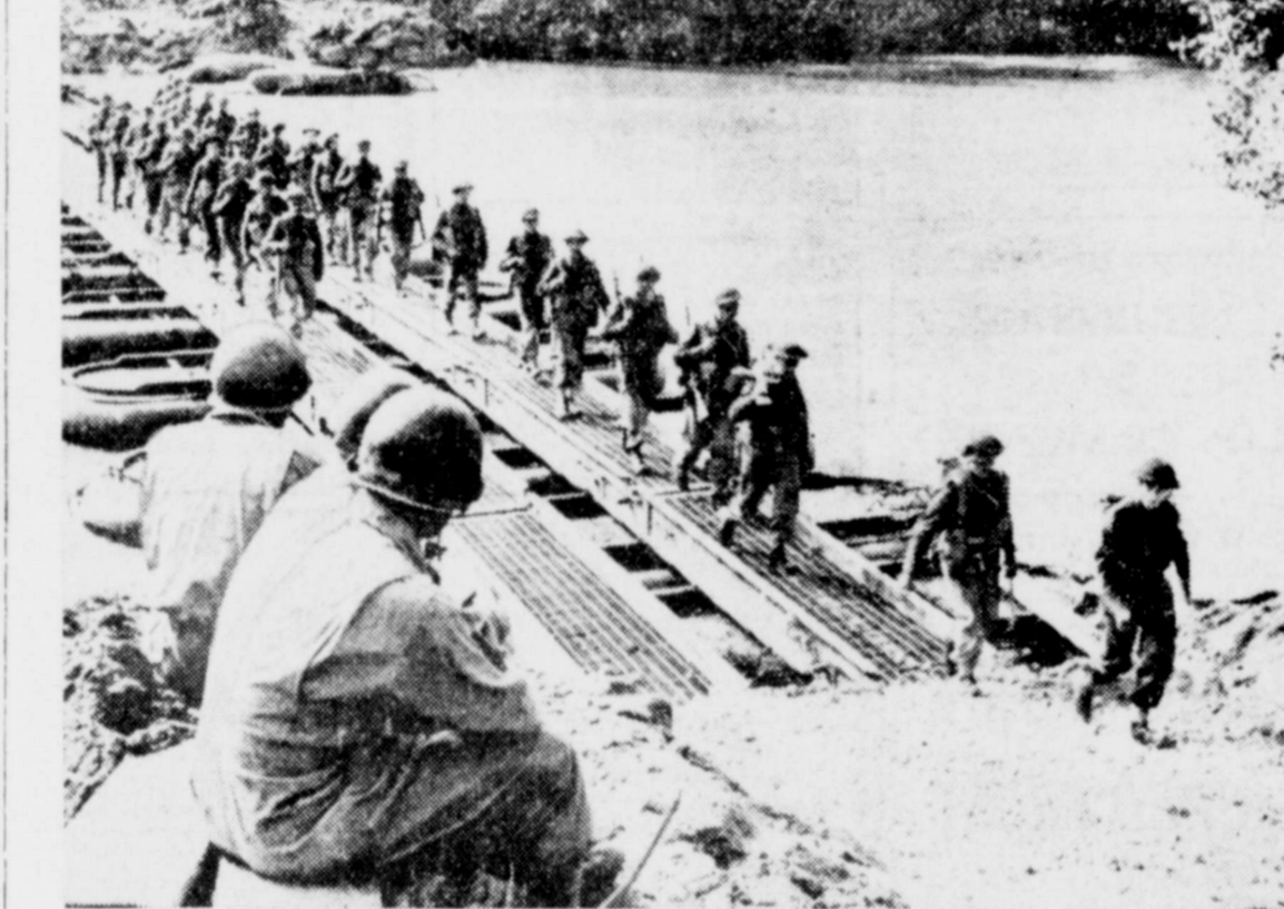
BRITISH TRY YANK BRIDGE—Three U. S. Army Engineers watch British troops cross pontoon bridge which Americans have just completed across Voltorno River, in Italy. Bridge was installed despite heavy fire by Germans, who tried in vain to hold position there and force Allies to withdraw. Germans themselves had to quit.
