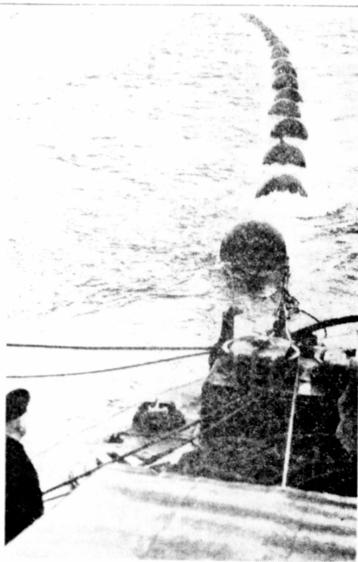
SUB NECKLACE —Nazi submarines still prowl about England's harbors, so stout nets are strung across port outlets. Here a Boom Defense ship tows this fancy "necklace" to the boom, to keep out would-be intruders.
