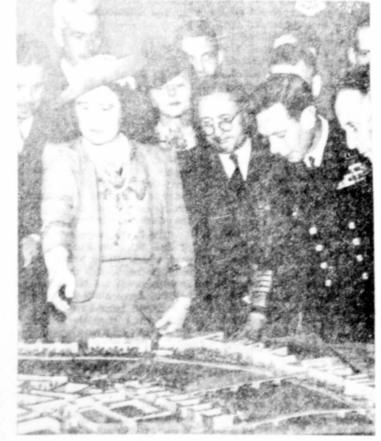
A NEW CITY—Britain's King George and Queen Elizabeth inspect models in London designed for rebuilding of British capital city. Models were on display at County Hall. Many Britishers think Nazi devastation was left-handed blessing.
