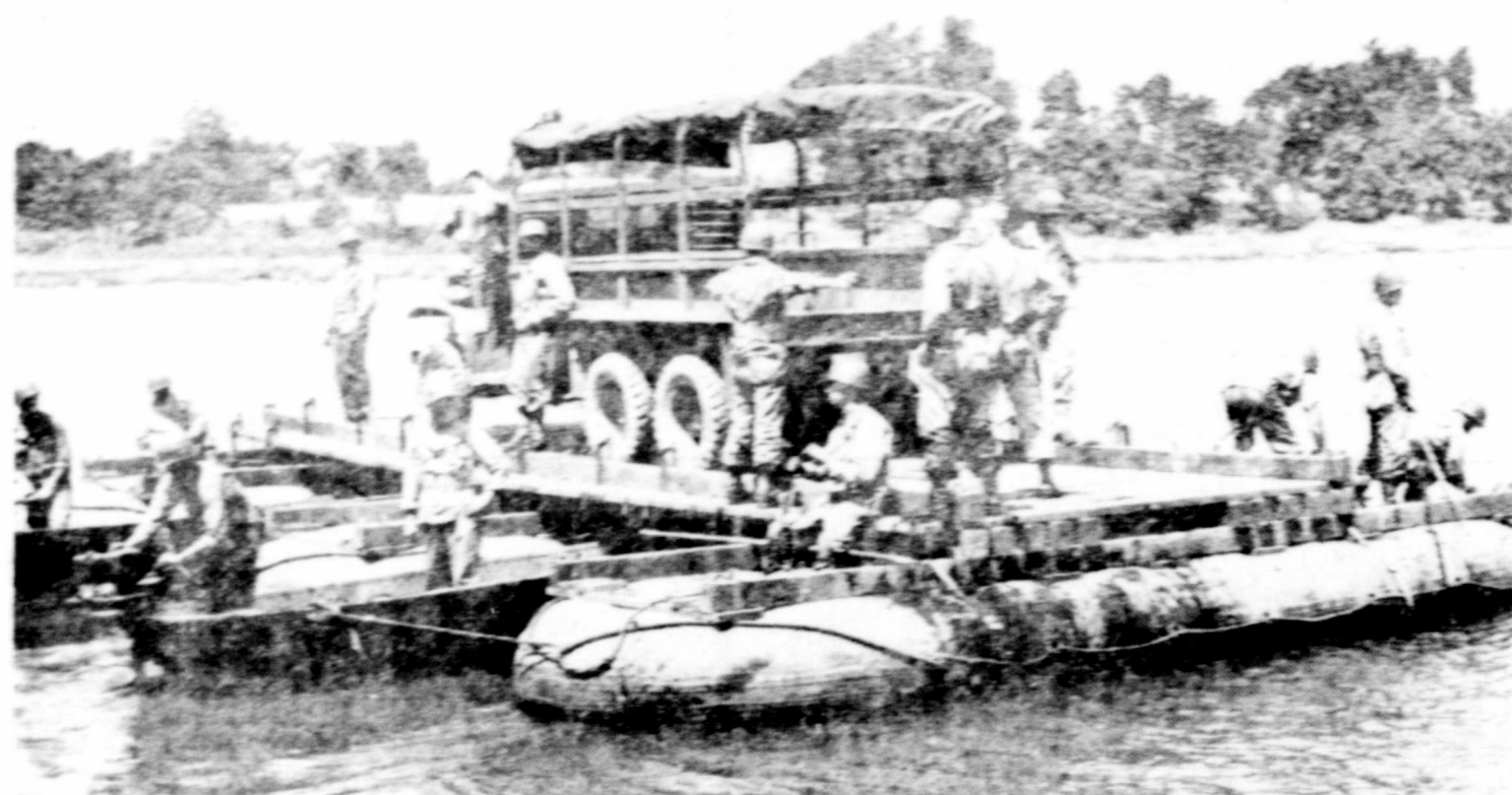
READY-MADE FERRY —Sometimes the Army wants to go where it wants to go, in a hurry. So it sends for the Engineers. They build the go-ahead out. Here's how they carry an Army truck across water on a pontoon bridge ferry. Demonstration of Engineer equipment was held recently in New York. It was shown the ferry could be towed almost anywhere.
