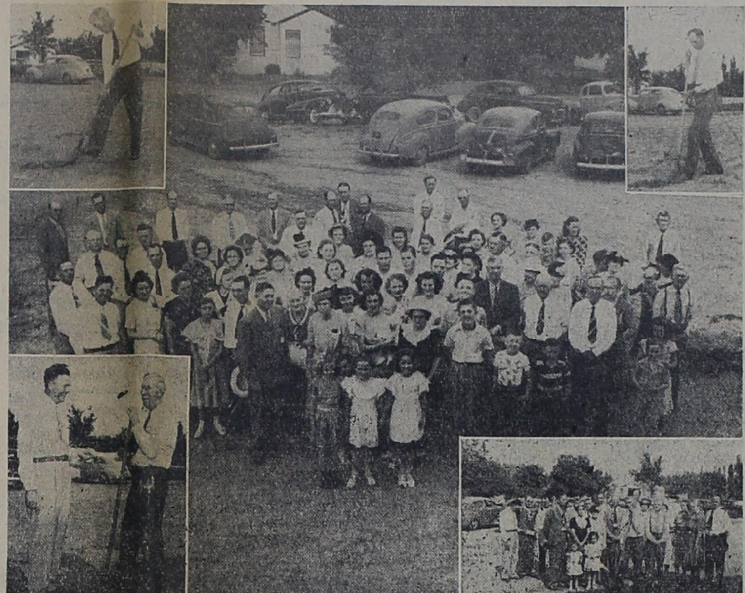
Pictured above are scenes from the ground breaking ceremony at the Baptist church Sunday afternoon when the $86,500.00 auditorium building program was officially launched. In the upper left corner is Kenneth Turner and in the upper right corner is J. O. Ayers, as they broke the first ground for the new building. Pictured in the center is a part of the congregation present for the services. In the lower left corner Lester Gladden is presenting Kenneth Turner, church treasurer, with a check to be applied on the building fund. In the lower right corner are some of the oldest members of the church along with special committees, including the building committee. The church building contract was awarded to the Clynch Bros. Construction Company of Childress.
