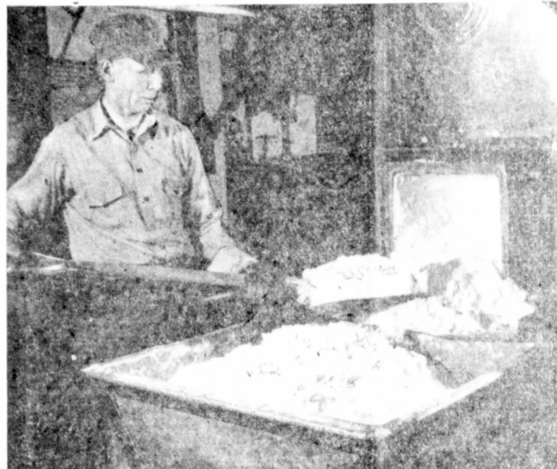
BLOCK-BUSTER'S STUFFING —White, crystalline substance that looks like granulated sugar is what makes the block-buster bombs do their jobs. It's called hexamine, made from formaldehyde and ammonia, at Perth Amboy, N. J., plant of Du Pont Company Workman is taking it from evaporator where it entered as liquid.
