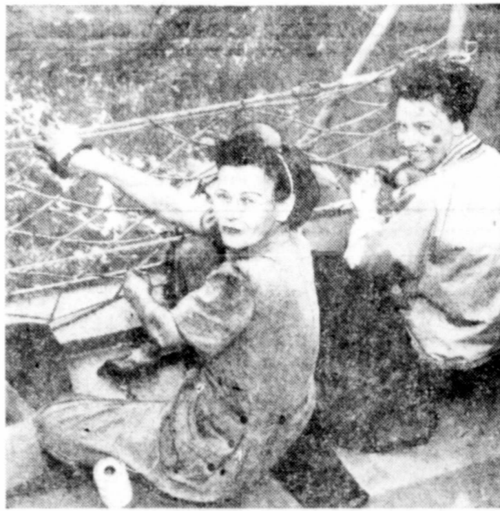
SAFETY WEAVERS —Using waxed cord, Vera Haddy, left, and Mary Early sew fast to rail of new destroyer escort, at Federal shipyards, Kearny, N. J. Life nets that will prevent men wounded or felled by high seas from being washed overboard.
