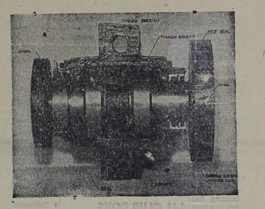
1. Two TIMKEN roller bearings to carry thrust. 2. DOUBLE SEALS at each end to seal out the dirt and seal in the grease.
