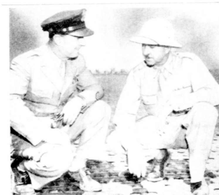
FOR DAKAR PLANES—Colonels Clifford Henderson, left, Los Angeles, and William N. Todd, Jr., Leavenworth, Kan., inspect section of steel runway newly laid at airport, Dakar, French West Africa.
