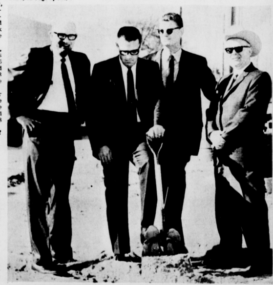
GROUNDBREAKING CEREMONIES--Alex Williams, left, Don Harmon welding the shovel, Marshall Cook and Jack Young were all present for the groundbreaking ceremonies Wednesday morning to begin the work for an addition to the Muleshoe Nursing Home. The new addition is expected to be completed early in 1969.
