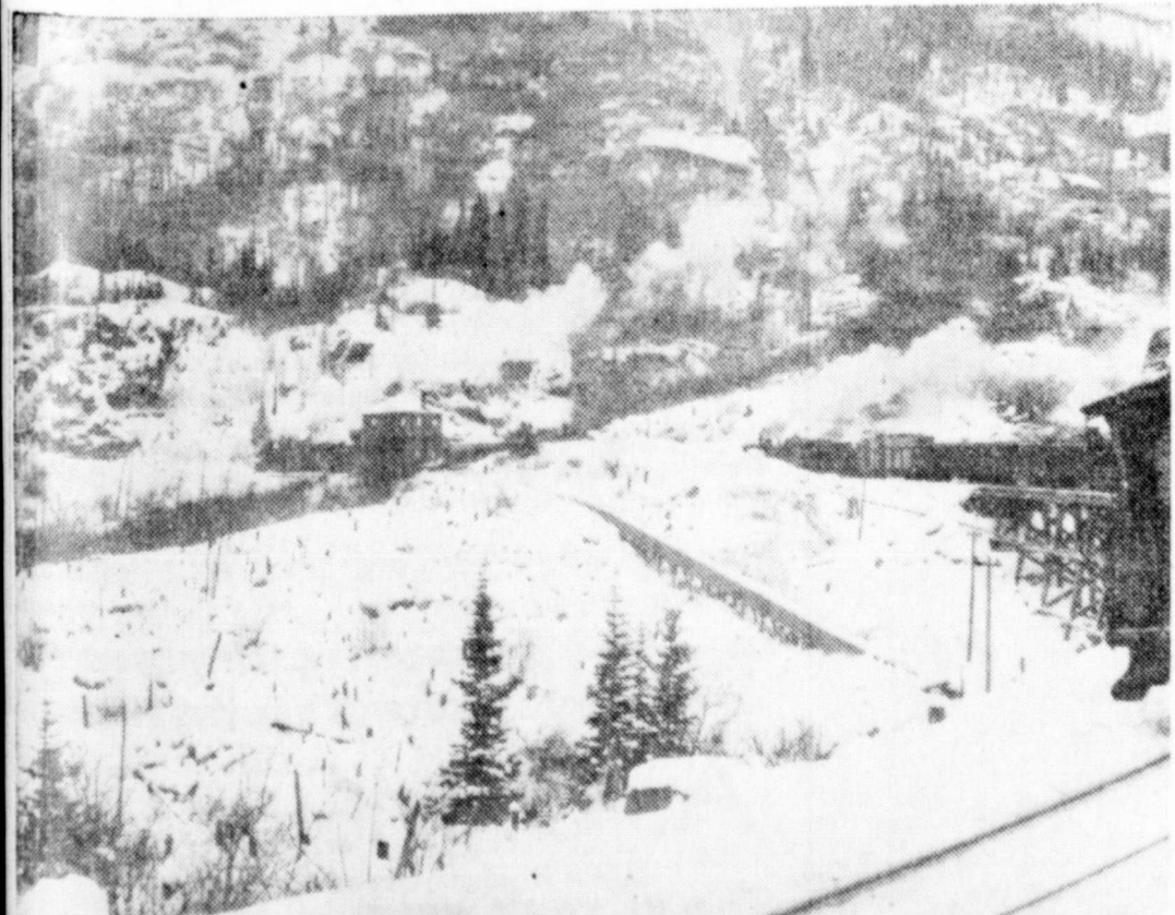
TOUGH GOING—Three engines are required to haul a load up the slopes of Alaskan Yukon Mountains, the only connection between the Alcan Highway and the Pacific ocean. Line was built some forty years ago to tap the gold fields of the Klondike. Doughboys operate the line.
