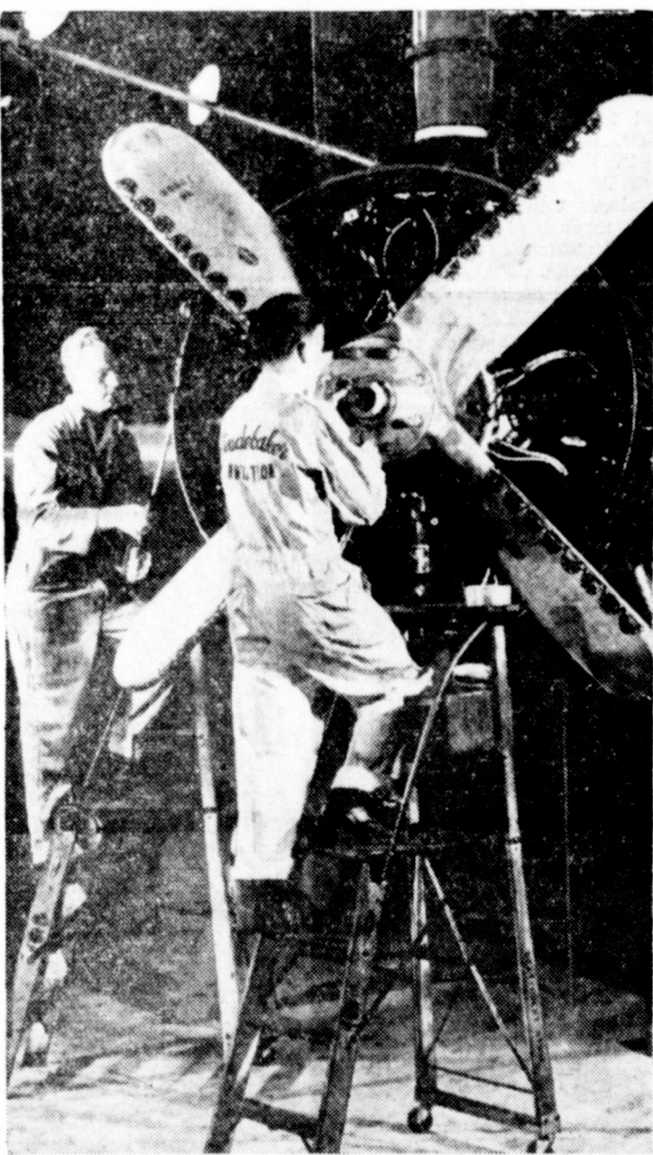
TESTING A "CYCLONE"—Mechanics make final checks on Wright Cyclone engine at Studebaker plant in South Bend, Ind., before starting on crueling test runs. (Passed by Censor.)
