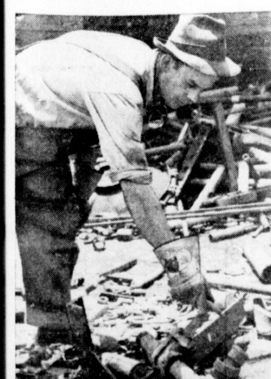
THE VALVE STANDS OUT AS USABLE.
