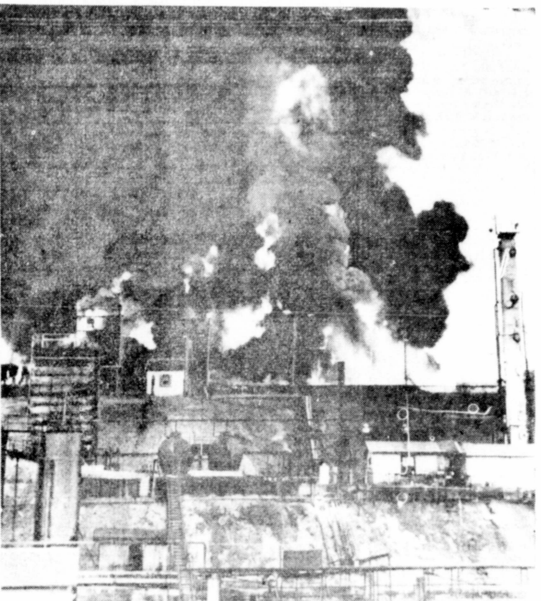
STATIC ELECTRICITY IGNITES OIL —An estimated 20,000 barrels of oil went up in smoke as flames roared through the Casimira Oil Refinery near Santa Maria, Calif., following an explosion which killed one worker and caused upwards of $50,000 damage. Static electricity was cause.
