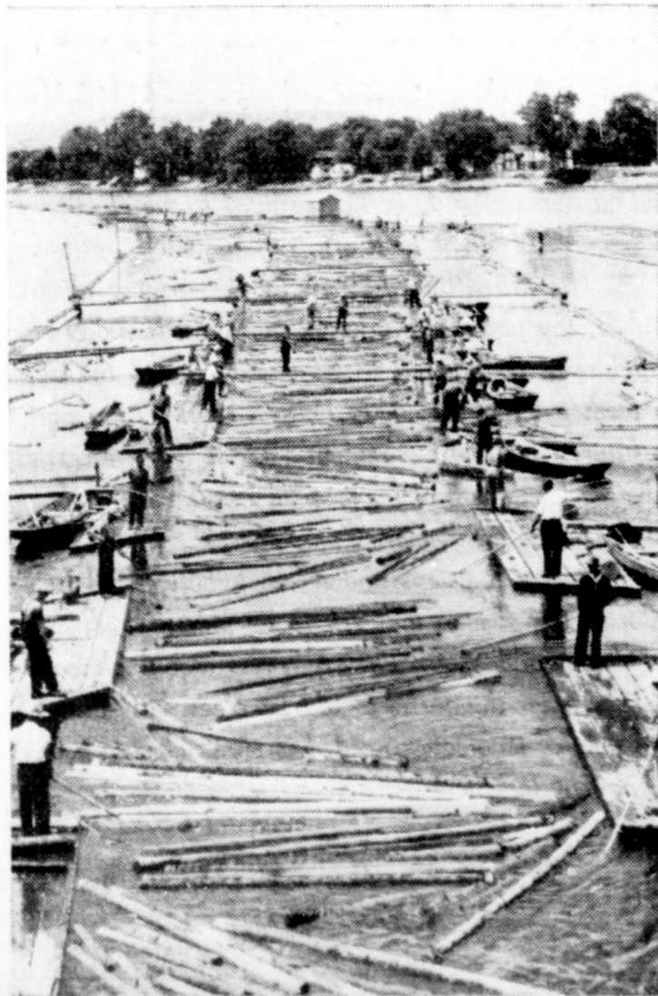
TIMBER ARRIVES AT DOWNSTREAM MILL.
