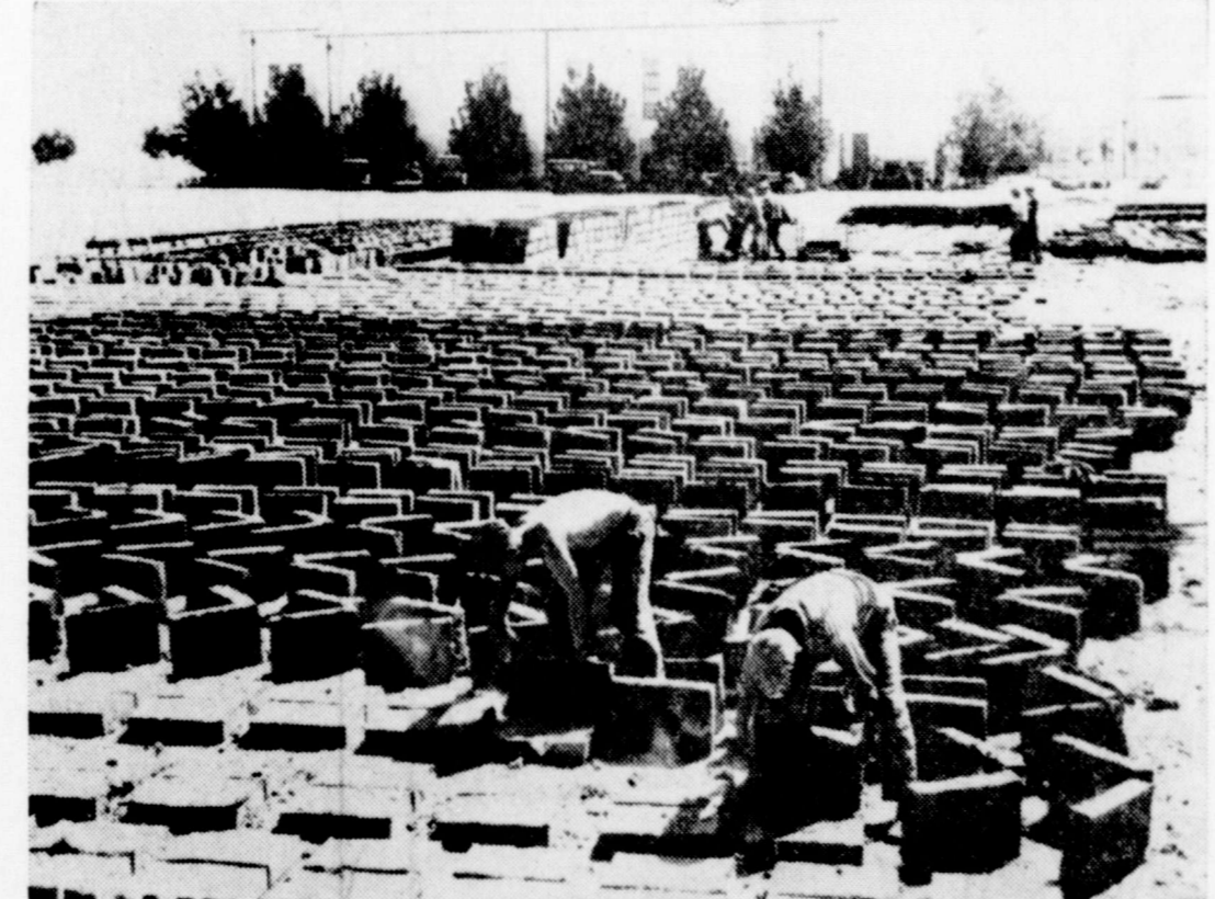
THE SUN DOES ITS PART AS BRICKS ARE LAID OUT TO BAKE
